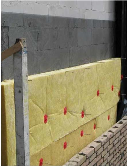
**Fig.6.** Brick wall construction and filling: (from left to right): white calcium blocks, G-ES netting, mineral wool insulation, 4 cm space, outer brick wall layer.
