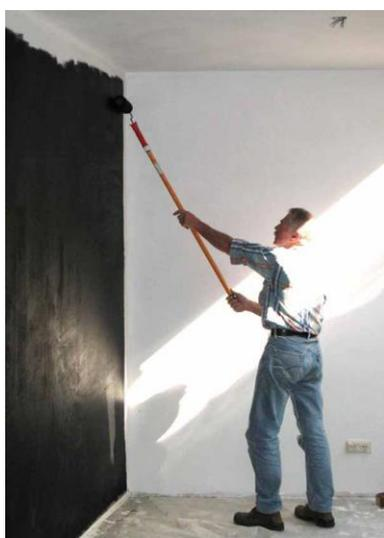
**FIG. 10.** Painting the wall black with two successive layers of Caparol, using a roller brush.
