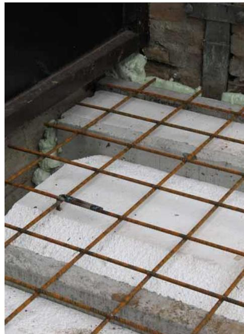
**Fig. 9** Reinforcement of concrete floor with steel mats, welded together at some points. Note that small piece of rod pointing downwards for an earth connection, if so
