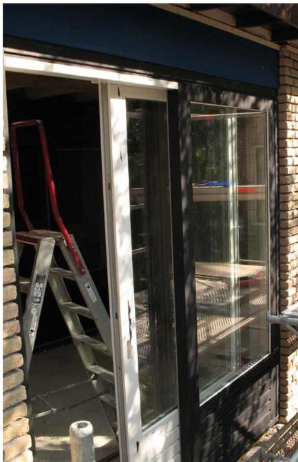
**Fig. 8** Treatment of wood with HSF54 paint. Two solid layers (one of the sliding doors) are next covered with two finish layers (not shown yet).
